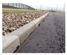
Infiltration trenches are stone-filled reservoirs to which stormwater run-off is directed, and from which the water gradually infiltrates into the ground. Their longevity is enhanced by incorporating a filter strip, gully or sump pit to remove excessive solids at the inflow. Filter drains (sometimes known as French Drains) are widely used by highway authorities. They are similar to infiltration trenches
